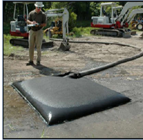
Plate 3-2. Silt Bag under inspection.
