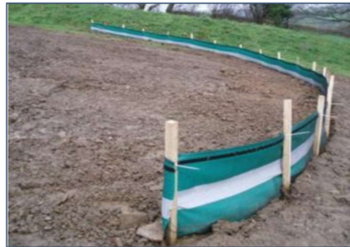
Plate 3-4 Embedded Silt Fence.
