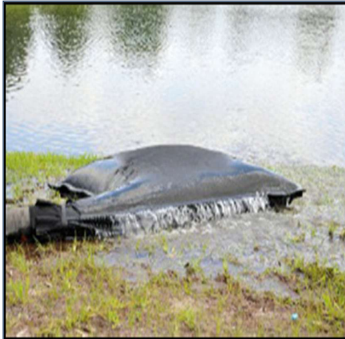
Plate 3-1 Silt Bag with water being pumped through.
